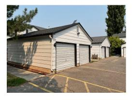
The siding in this area is a fiber board wood based siding. This item is in very poor condition and should be replaced very soon to avoid damage to the building structure. The garages are not included in this reserve item due to budget constraints. Garage siding replacement is included in another item.
