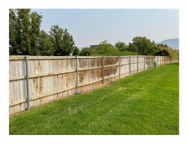
Replacement of wood perimeter fences. This includes the fences along the perimeter of the property along with the outside fences on the patio of each building. It does not include partition fences between each unit. The condition of the fences varies greatly because some fences have been replaced by the owners and other have not.
