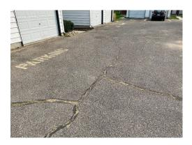
Asphalt should be sealed on a regular basis to prolong the life of the asphalt. This item had been deferred until such time as the asphalt is replaced. The asphalt is failing and will need replacement soon to avoid major parking lot damage such as potholes, alligator cracking and damage to the base.
