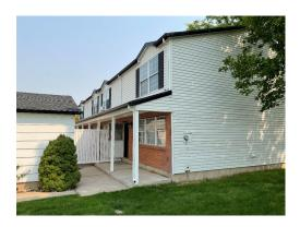
The siding in this area was replaced on the townhomes in 2019. The garages were not done at the same time and are included in another reserve item. Replacement of the fiber board wood siding with vinyl siding is projected.
