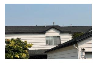
The roofs are an asphalt shingle in the architectural style with a manufacturers estimated life of about 30 years. In the Utah climate the life of this component is reduced to about 25 years. This component has been replaced over the past 13 years but for this report we have split the replacement into two phases. Cost estimates are based on actual replacement cost in 2020 that were necessary due to wind damage.
