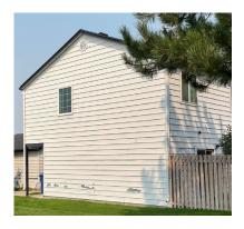
The siding in this area consists of two buildings with metal siding and one building that has vinyl siding. The metal siding is in need of new paint but the siding is protecting the structure as it should. The garages are not included in this reserve item due to budget constraints. Garage siding replacement is included in another item.
