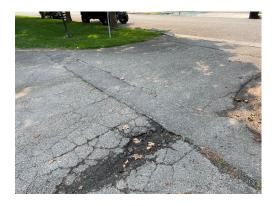
The asphalt is in poor condition and is in need of replacement in the near future. Replacement cost estimates include removal of existing asphalt and replacement with 3 inches of new asphalt. It is assumed that the base material in in good condition and will not need to be replaced. If it is discovered that the base needs to be removed and replaced this will increase the cost significantly.
