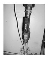
There are 2 water valves. The main is outside & requires a special tool to shut off. So, in case of any emergency that requires you to stop water flow into your home, use the valve shut off in the utility closet. Look for a handle on a copper pipe coming out of the floor & turn it to the off or horizontal position. This will stop water from entering your home pipes to that point.
