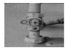
In case of any emergency that may cause a gas leak, locate the gas meter. It is usually in the front of your unit. Look for the valve shown above. **Use a crescent or box type wrench of the appropriate size and turn until the holes**line up.
