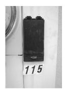
To turn off the power to your unit, locate the main box on the outside of the unit. Locate the small cover next to your unit number & switch it to off. This will stop ALL power to your unit. **Do only in times of emergency.**
